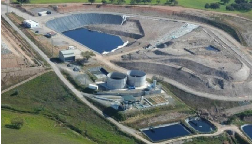
Image 2.1 Aruwakkalu sanitary landfill
