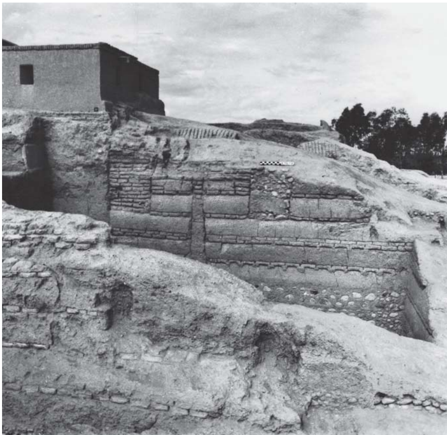
Fig. 6: Tape Šotor, room no. 57, view from east to west, showing the condition of the eastern wall of constructions 52–56, with the sealed windows against which terrace 57 was built.
