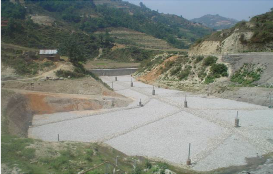
Figure 8: Sisdol landfill site before operation
