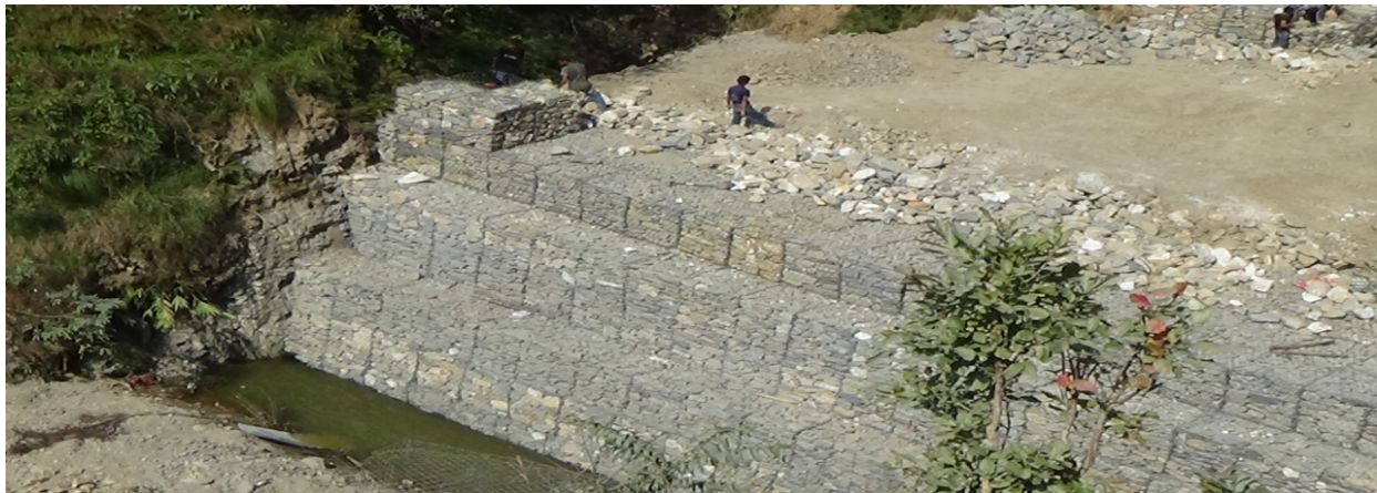
Figure 13: Construction site of new sanitary landfill site at Bancharedanda
