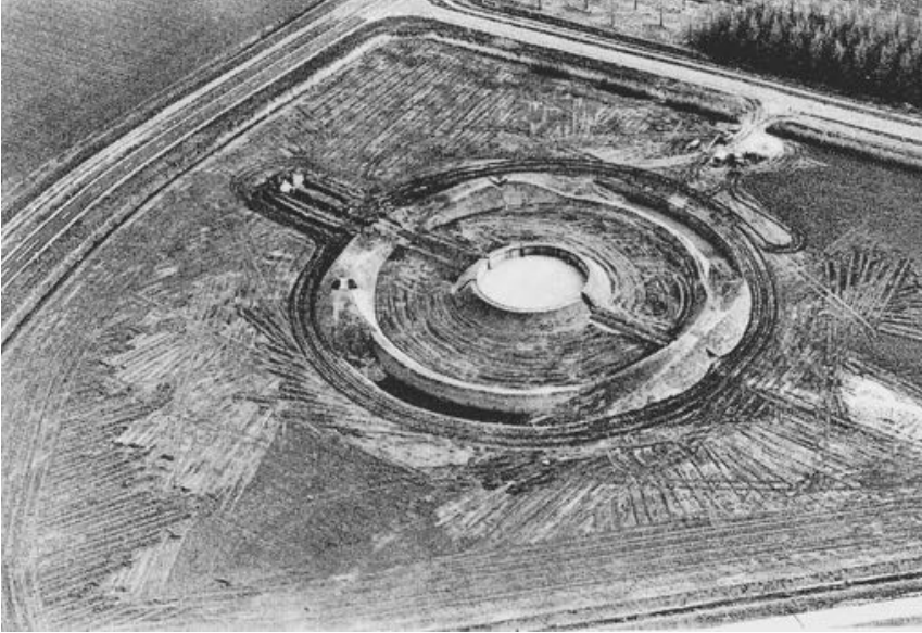
Figure 4.10. Robert Morris, Observatory , 1971/1977. Earth, water, wood, granite, steel. Diameter 298 ft., 6 \frac{7}{8} in. Oostelijk Flevoland. Photo: © 2021 Estate of Robert Morris/ARS, NY.
