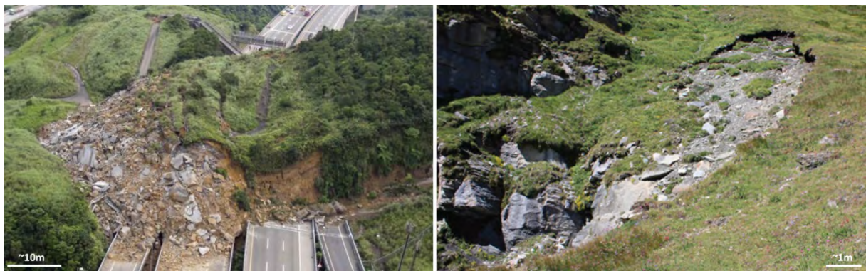
Figure 1.3: (Left) Large deep-seated landslide burying an entire Taiwan highway section (source: Metronews journal). (Right) Shallow planar slide affecting the first 30 cm thick layer of the morainic soil, in the Upper Bagnes valley.
