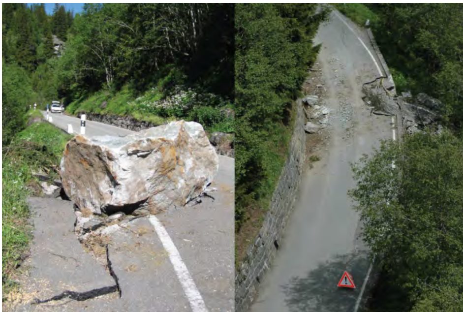
Figure 5.1: Photography of a rockfalls event in 2006 that reached twice the road section near Le Plamproz , in the Bagnes Valley.
