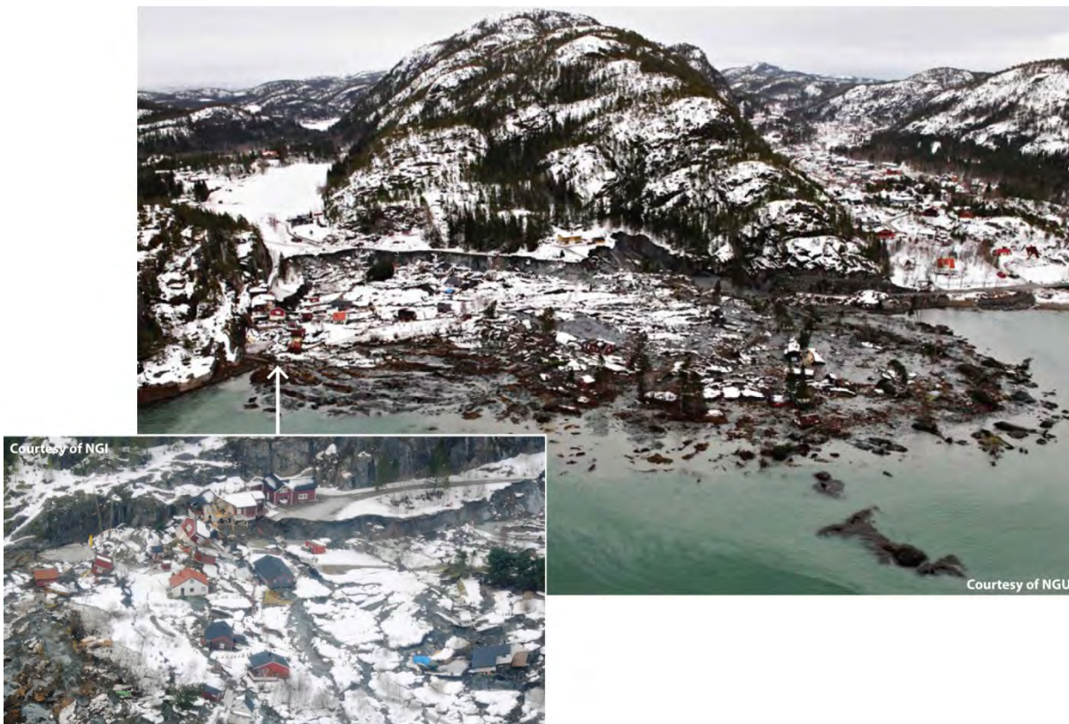
Figure 1.6: In Namsos, May 2009, a huge soft soil slide occurred just after blasting operations for road. Ten houses were destroyed but fortunately without making any fatality (pictures: courtesy of NGU and NGI).
