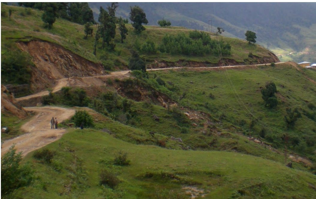
Figure 6.4: Cut and filled slope led to rotational earth slide along a Nepalese road in 2008 (courtesy of A. Breguet and K. Sudmeier-Rieux).
