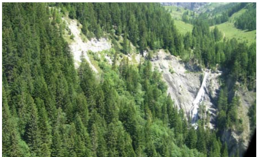
The water turn-out from the tunnel of Mont Lachaux on the Ertentse. © Emmanuel Reynard
