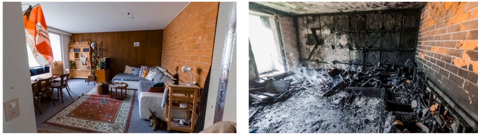
Fig. 2. Scene of Scenario 1. Before the fire (left); After the fire (right). Credits: Service Presse, Police Neuchateloise.
