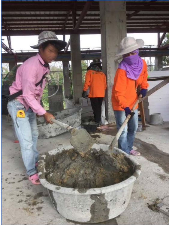
3A: Manual cement mixing
