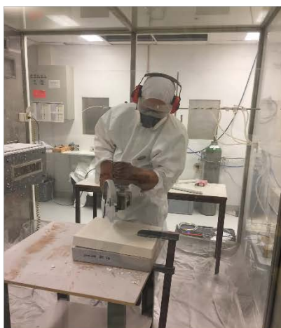
1B: Concrete cutting
