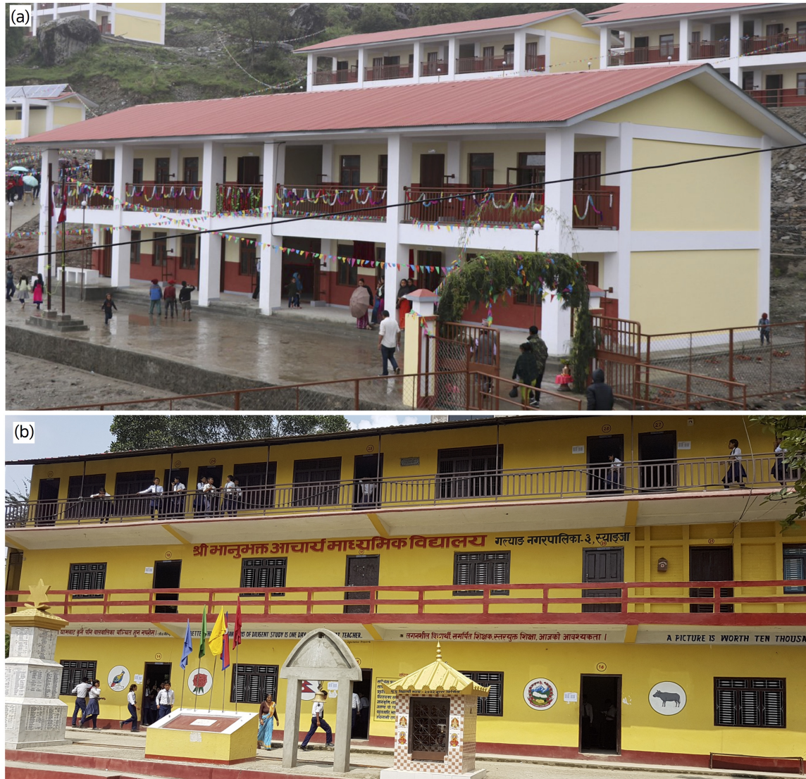
Figure 4.2: School buildings participating in our program. (a) Shree Himalaya Secondary School in Barpak, Gorkha district. A reinforced cement concrete (RCC) building was newly constructed after the 2015 Gorkha earthquake. A total of 672 students study in the school. (b) Shree Bhanubhakta Acharya Secondary School in Galyang, Syangja district. RCC building, but the third story is not cemented: it is brick, with tin roof on top. A total of 925 students study in this school.
