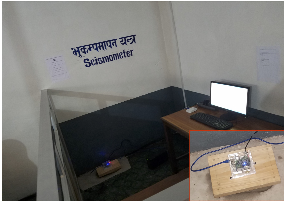
Figure 4.6: Example of the setting of an installed seismometer, in Shree Siddha Baba Secondary School, Gulmi district. The sensor is installed on the ground floor by making a partition in the Accounting Room; it is fixed to a wooden block which is itself fixed into a ca. 2 cm thick cemented base on the ground (inset). The station is connected to a desktop computer for real-time data visualization via the jAmaSeis (Drago et al., 2009) software. Detailed information on how to visualize waveforms on a smartphone using the EQInfo app is printed on the wall (A4 paper). The word “Seismometer” is written in on the wall in Nepali (and English) language.
