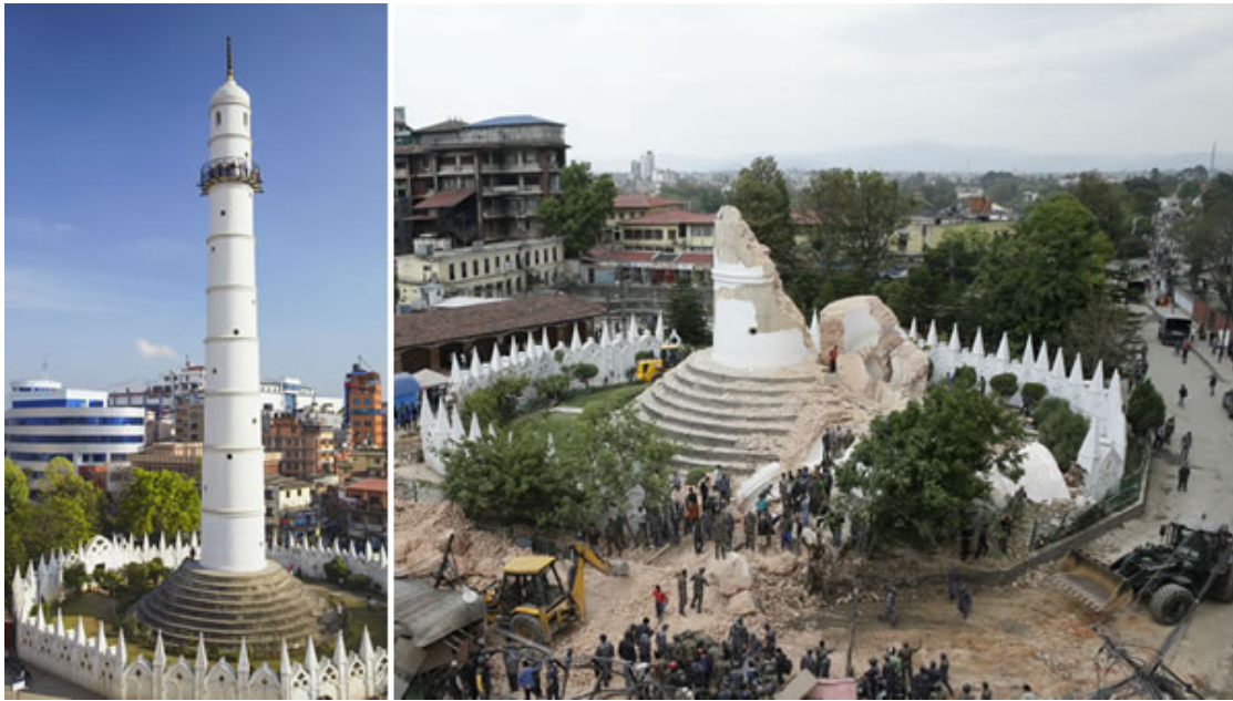
Figure 1.8: Historic Kathmandu tower ‘Darahara’ before and after the 2015 Gorkha earthquake. This is an example of brick/stones masonry building. (Courtesy: Narendra Shrestha, EPA).
