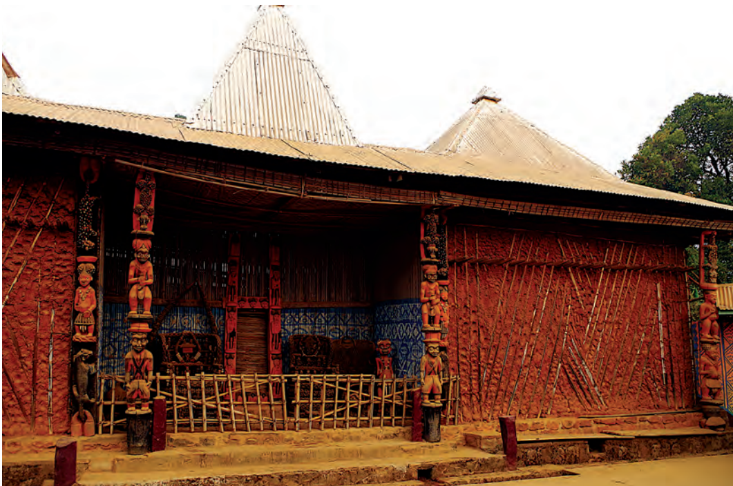
7. Palace of Oku chiefdom, partly constructed with Raphia petioles (bamboo). Elak-Oku, 2016. Photo by Thomas L.P. Couvreur.
