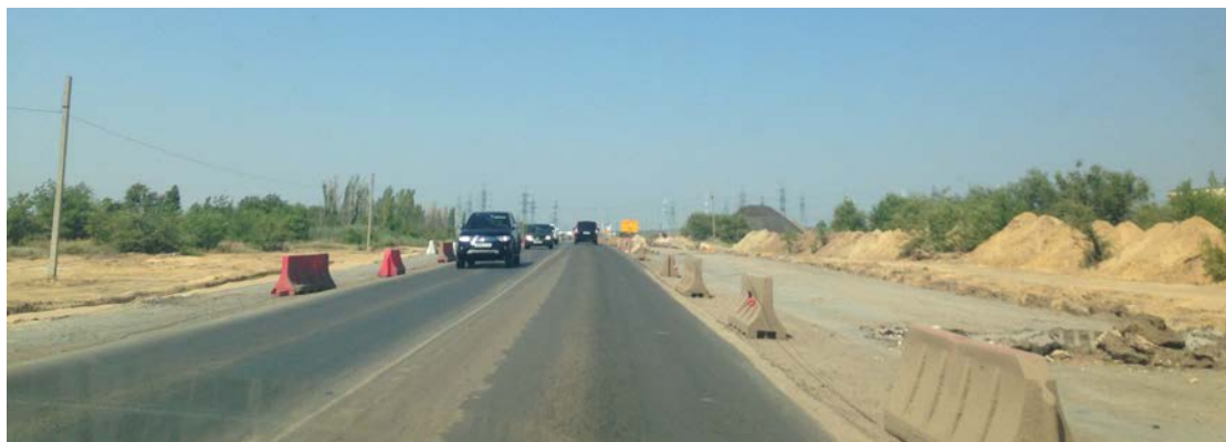
Figure 33: Volgograd Aviators' Highway under construction in 2016. At this point the expanded lanes had not yet been opened for use, but the newly repaved parts of the road were already cracking. Source: author.
