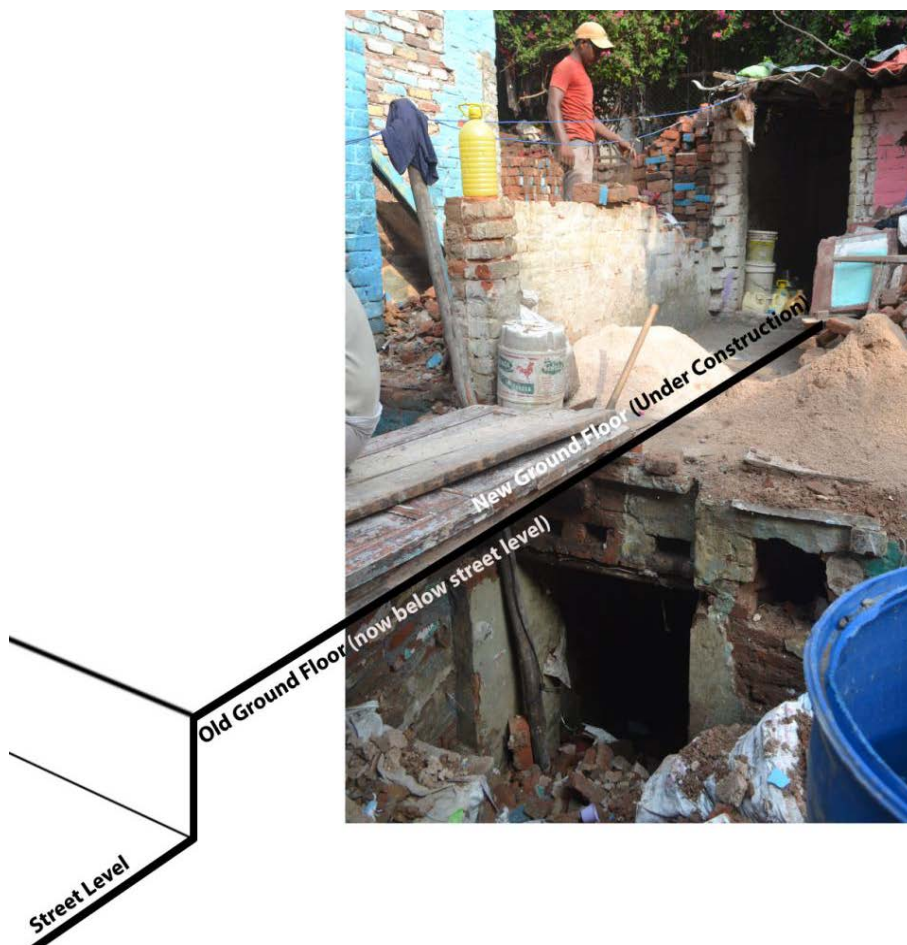
Figure 8: Sketch showing the ground floor being below the street level in Jagdamba Camp (© Author)
