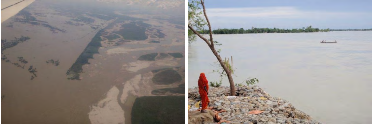
Figure 97. Left: Koshi River dyke breach seen from airplane; right: Point along dyke where breach occurred. September, 2008.
