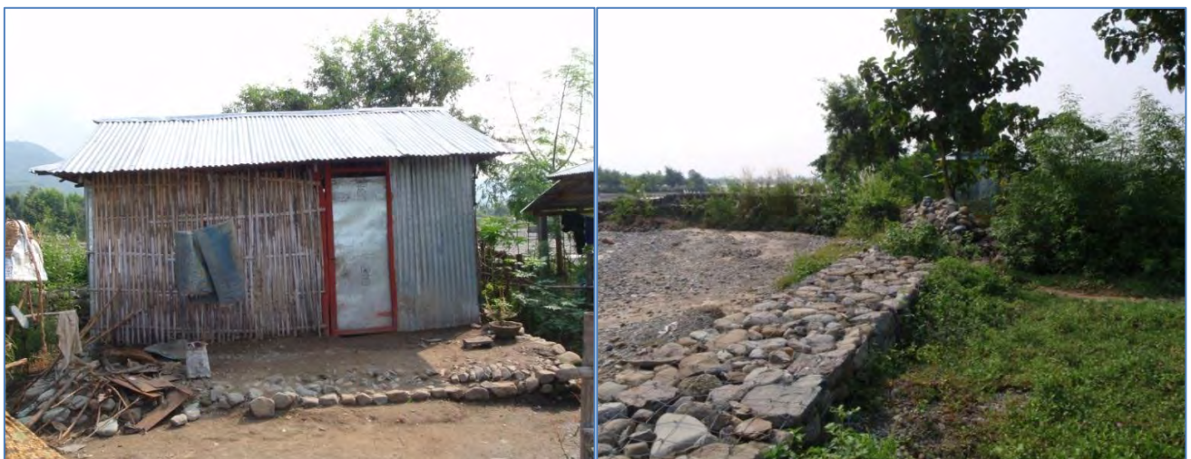
Figure 125. Top left: Google Earth image, 2004 of Seuti River. Top right: Same river bank in 2009 (GeoEye, 2009) with new unplanned settlement in the riverbed. Bottom left: House with three family members living by Seuti Khola; Bottom right: gabion wall along Seuti Khola, September, 2009.
