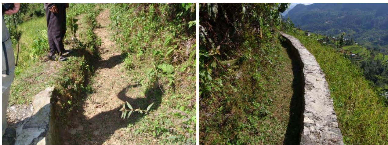
Figure 79. Left: cemented irrigation canal. Right: partly cemented irrigation canal, October 2010.
