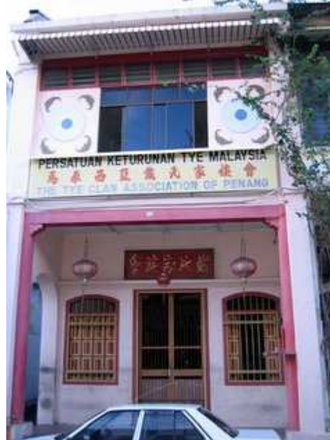
Figure 12. A shop-house, George Town (authors' image)
