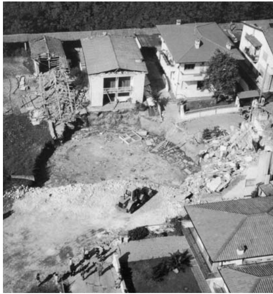
Figure 1.3: Example of catastrophic sinkhole in the Italian municipality of Camaiore, in Tuscany (Picture by L. Micheli from: Buchignani et al., 2008 ).
