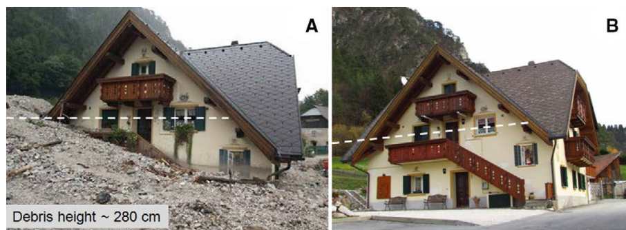
Fig. 5 Building impacted by debris flow (A) 1 day after the August 2003 event and (B) during the field work campaign in 2013
