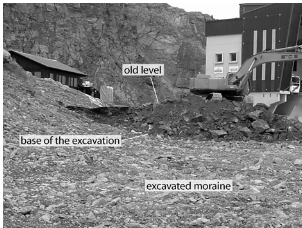
Fig. 3. Excavation works carried out in October 2006 to the south of the cable car station, on the road leading to the glacier.
