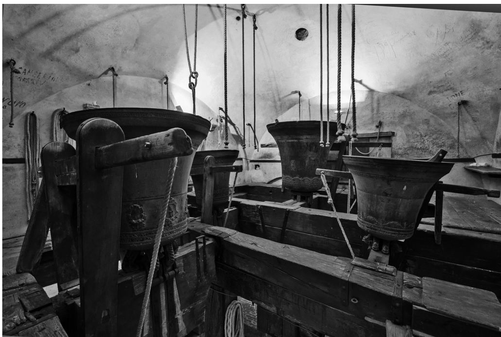
Fig. 3: Bells of Bologna Cathedral (Italy). Between two subsequent peals, bells can be left in the “up” position by shoring up the bells with special beams.
