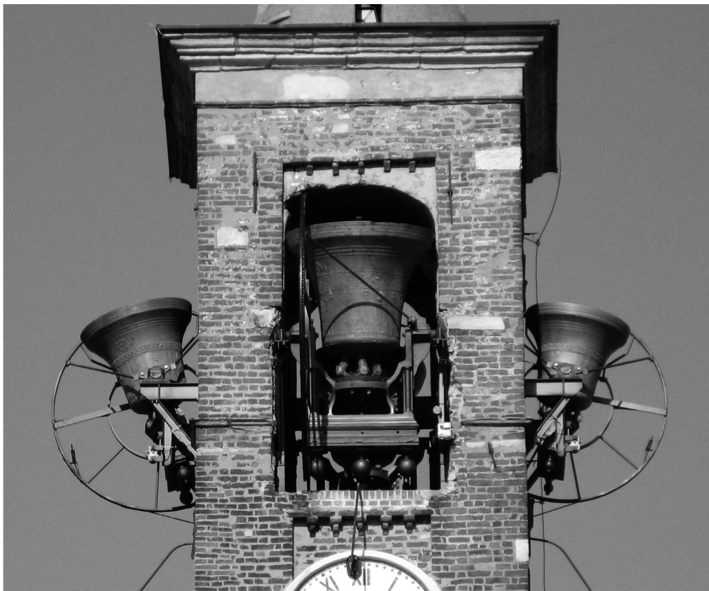
Fig. 5: Bells of Santa Maria del Cerro in Cassano Magnago (VA – Italy) in the “up” position during a motorized concerto peal (photo by Roberto Luigi Botta). The heavy counterweights reduce the forces acting on the structures and allow big bells to be hosted in small towers.
