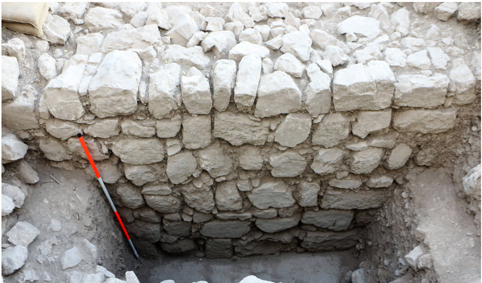
3 Two construction methods in the support wall in the southeast of the site: the lower courses, established on bedrock, were built of large boulders, while the upper courses were constructed of medium-sized, square-cut stones (Courtesy of the Shmunis Family Excavations at Kiriath-jearim)
