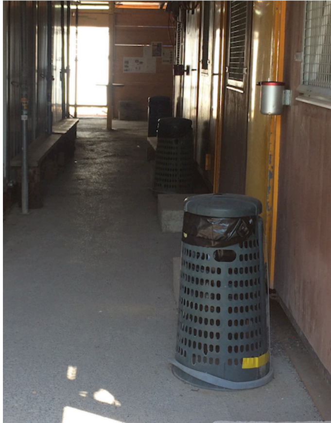
Figure 19: The trash bins at the construction site were made of plastic and had holes. The lids had to be opened by hand and were sometimes left open or blown open by the wind. (source: author)
