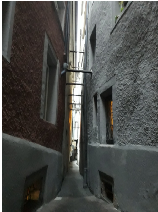
Figure 14: A narrow alley in the Old Town of Zurich. The buildings are several hundreds of years old and require to be stabilised by horizontal bars. Renovation is difficult and often very costly due to challenges of lack of space, uneven terrain and weak foundations of the underground. (source: author)
