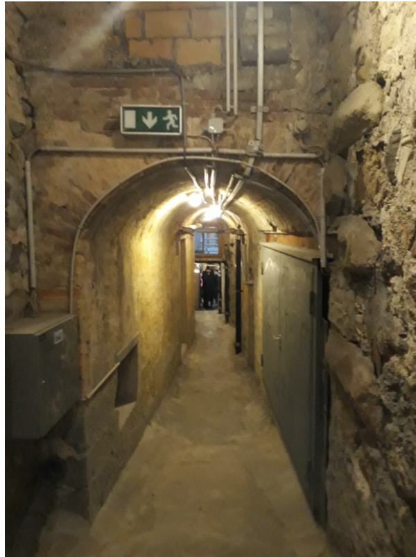
Figure 15: The old town of Zurich has buildings that are several hundred years old. The sewage system is also old and suffers from pipe breaks and leakages. As buildings are renovated, the sewage pipes are upgraded too. (source: author)
