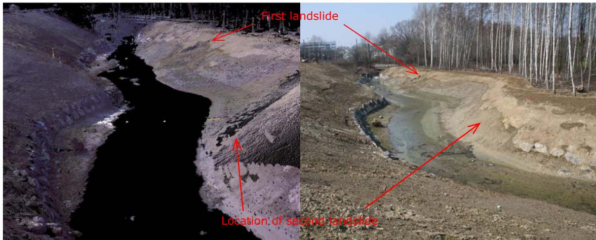
Figure 1: Views of the Sorge River to the West (taken on March 16<sup>th</sup> 2006). The point cloud of the laser scanner and the photograph show the area of the remedial works that were done in 2005. The scar of the first landslide is also shown.
