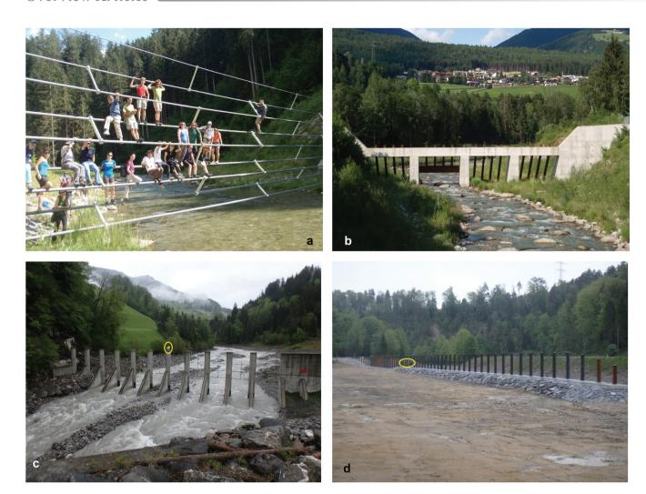
Figure 6. Examples of structures used to limit downstream mobility of wood. (a and b) Rienz River, Italy; (c) Chiene River, Switzerland (the chair is outlined in yellow for scale); (d) Sihl River, Switzerland (people are outlined in yellow for scale). The structure on the Sihl River is unique in size and design. It is installed parallel to the flow in the outer bend of a meander to retain wood (which might otherwise reach the City of Zurich) but to allow sediment to be transported.
