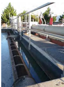
Figure 3 UAF test unit (from left to right: inlet, test unit, compartment volumes)
