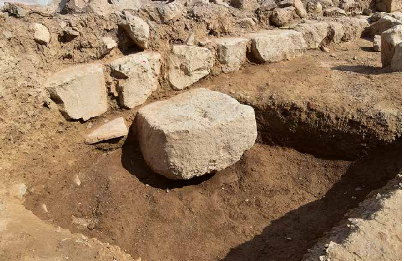
Fig. 15. Limestone base under east wall of edifice 3 (St21)
