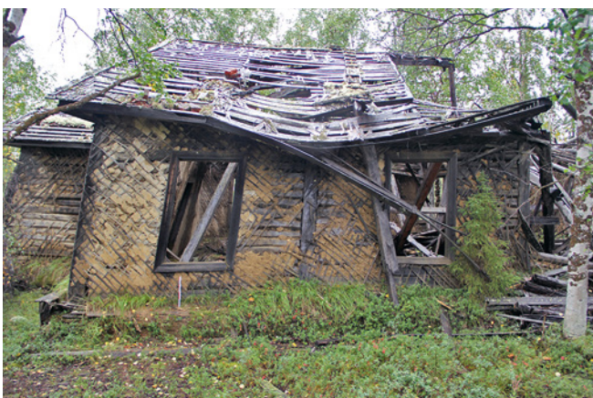
Figure 6. External wall of barracks B5 (J. André).
