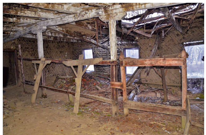
Figure 8. Interior of the eastern dormitory of barracks B5 (J. André).
