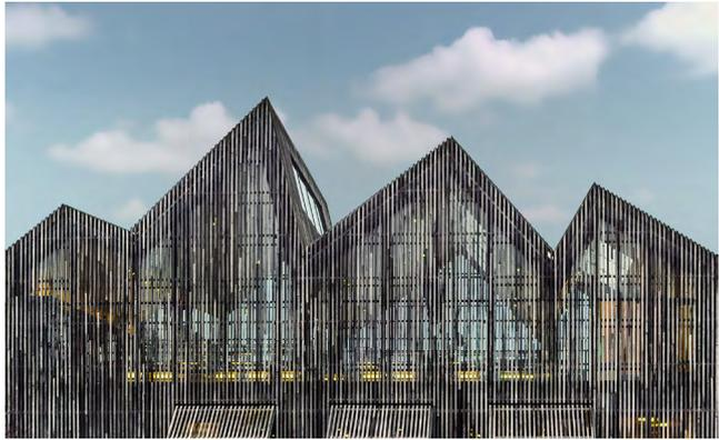
local tradition of beachcombing and recycling. Indeed, like many of the objects exhibited in the museum, these cladding elements also come from the sea – in this case sawn hardwood sheet piling recovered from the North Holland Canal and given a “second” life in the building [Fig. 3].
