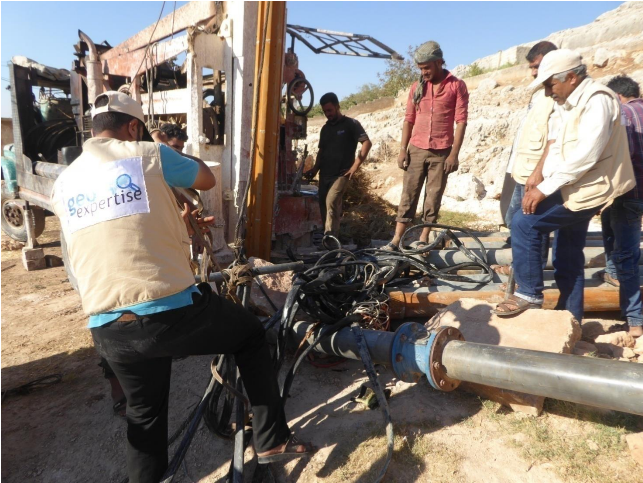
Figure 6.2. 13: Restoration of the wells (Photo, Geo Expertise, August 2017)
