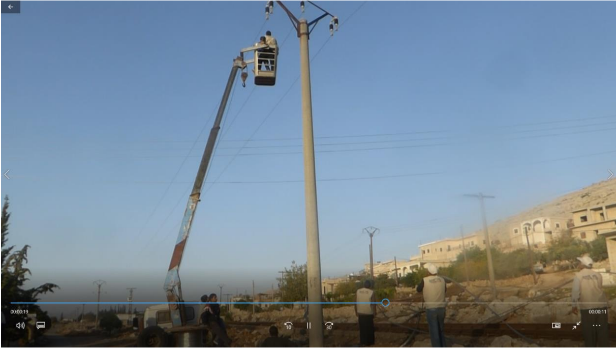
Figure 6.2. 16: Repair of electric network, (Photo, Geo Expertise, February 2018)
