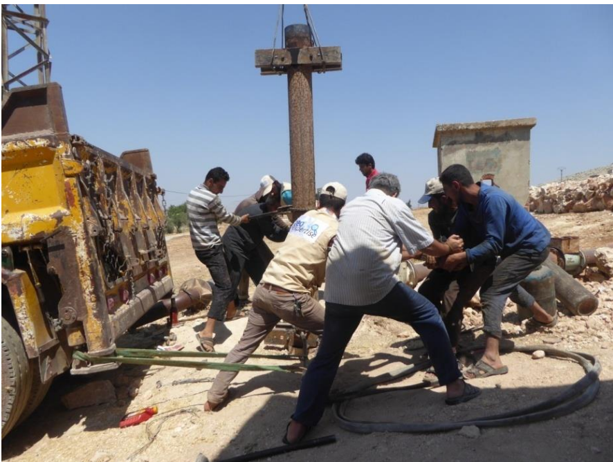
Figure 6.2. 14: Repair or replacement of pumps (Photo, Geo Expertise, August 2017)
