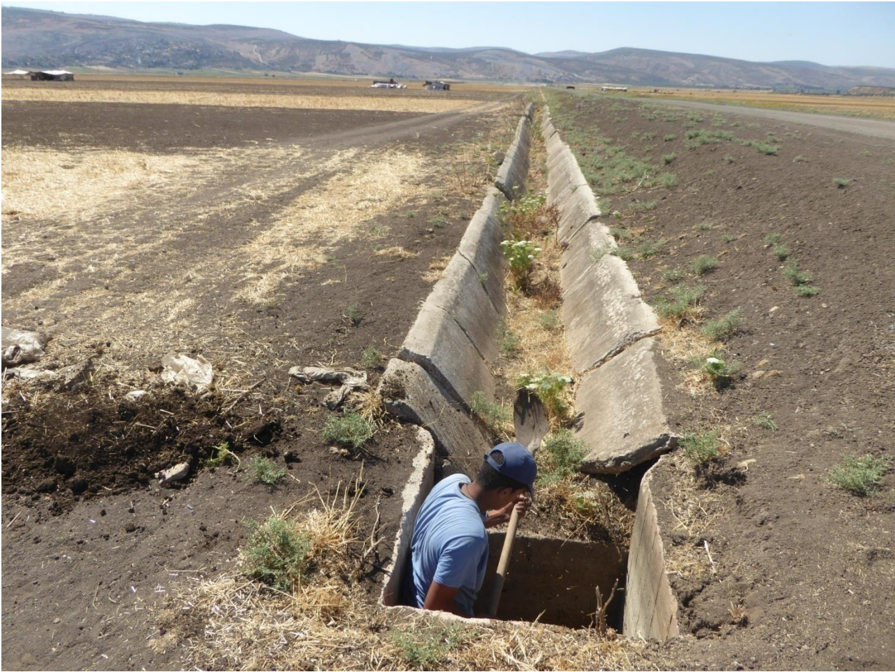
Figure 6.2. 10: Clean inspection room ( Photos, Geo Expertise, June 2017 )
