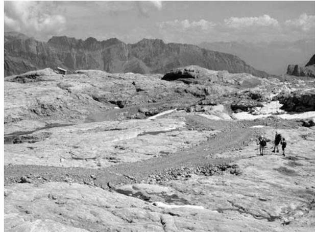
Fig. 7- An illegal road built on the karst of Tsanfleuron (Valais, Switzerland) by extracting gravels from a Little Ice Age morainic crest. The road is now dismantled and the moraine recovered after an EIA performed a posteriori.
