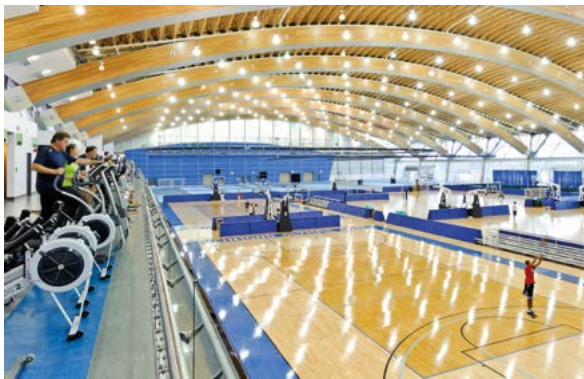
Richmond speed-skating rink built for the 2010 Vancouver Games, which won several prizes for its advanced environmental design and which is used today for several sports other than the speed skating for which it was used during the Games
