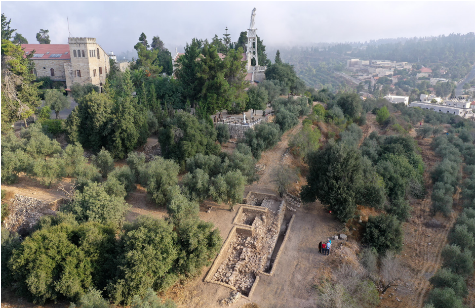
FIGURE 7 Area B, looking north; note that the massive wall exposed in Sub-Area B1 continues under the big north–south terrace which delimits the summit of the mound in the east.
