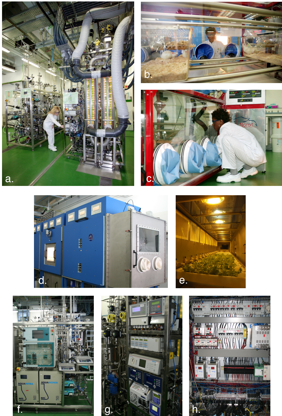
Figure 7: Le MELiSSA Pilot Plant (MPP).
