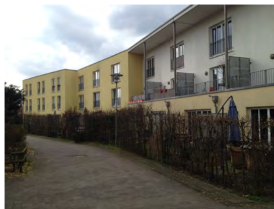
Photo 51: Western part of the row houses in Weißenburg
