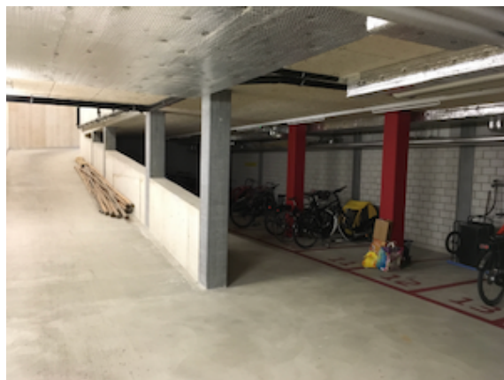
Photo 16: Underground bicycle parking and drivable access ramp in Giesserei
