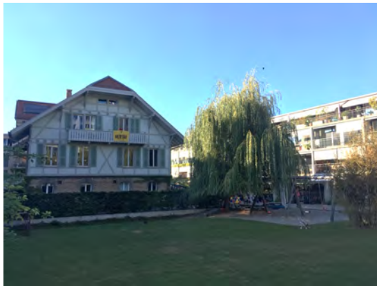
Photo 2: Half-timbered house with nursery, common room and dwellings in Burgunder
