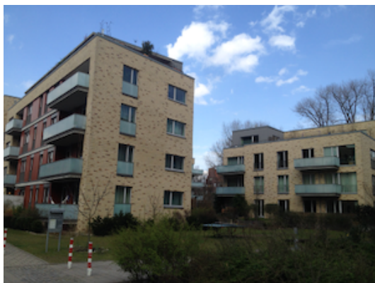
Photo 37: Most recent part of Saarlandstraße
