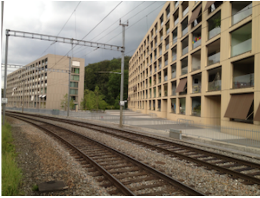
Photo 24: The two buildings of Sihlbogen
