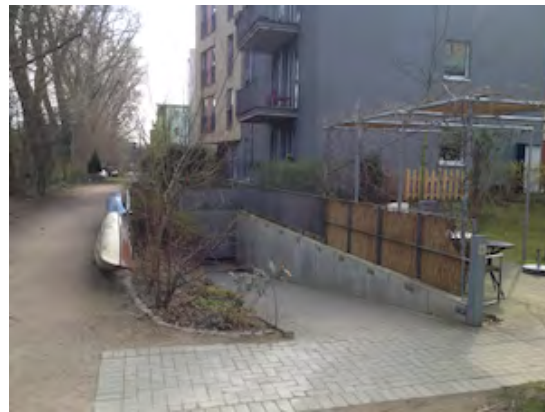
Photo 39: Drivable ramp to bicycle parking
