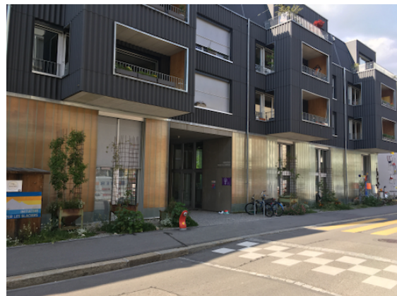
Photo 8: FAB-A seen from the outside, with live-in studios on the ground floor
