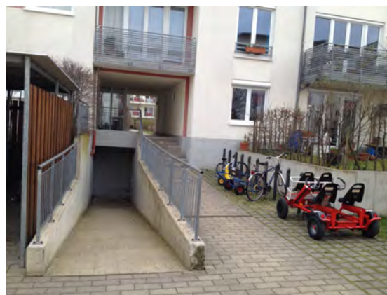
Photo 47: Drivable ramp to bicycle parking and outdoor bicycle parking space for short-time parking
