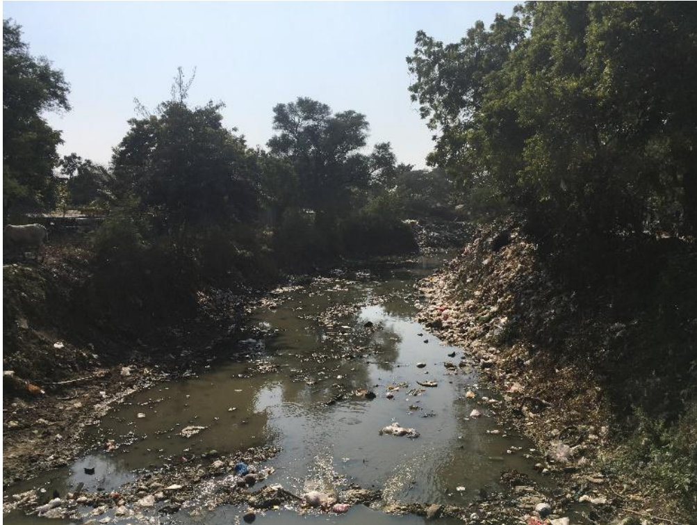
Figure 6. Unlined drain in Pyi Gyi Tagon. Source: J.Sanchez
